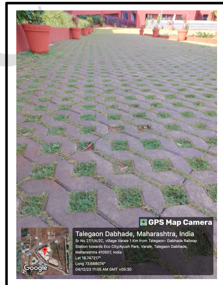
Grass Block Pavement Walkway at Dr. D. Y. Patil College of Engineering & Innovation
