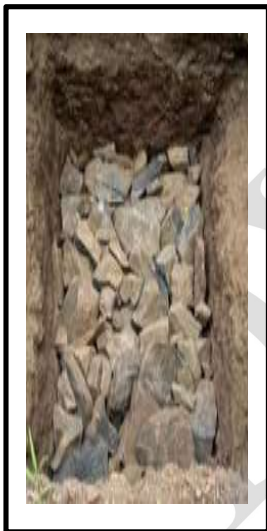
Material Filling in Pit
