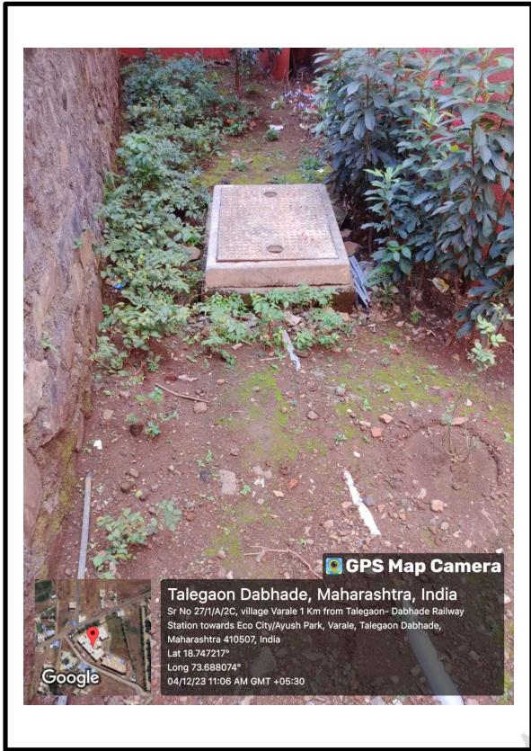
Pits Connected to roof top water for ground recharging.
