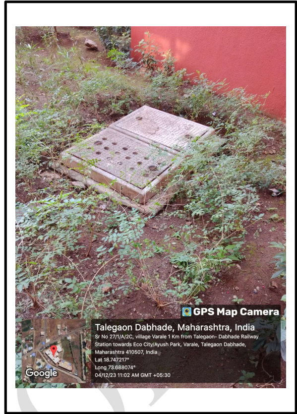
Pits Connected to roof top water for ground recharging.
